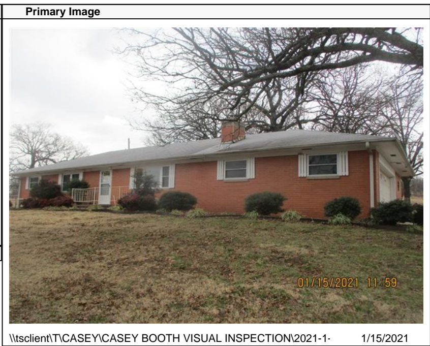
\\tsclient\TCASEY\CASEY BOOTH VISUAL INSPECTION\2021-1- 1/15/2021
