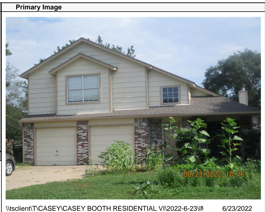
\\tsclient\TCASEY\CASEY BOOTH RESIDENTIAL VI\2022-6-23\ 6/23/2022
