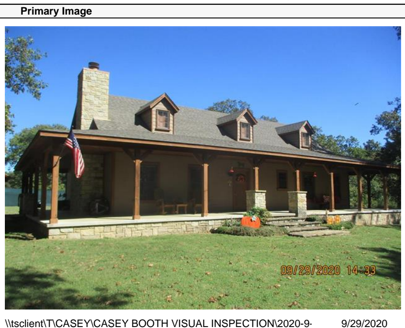
\\tsclient\TCASEY\CASEY BOOTH VISUAL INSPECTION\2020-9- 9/29/2020
