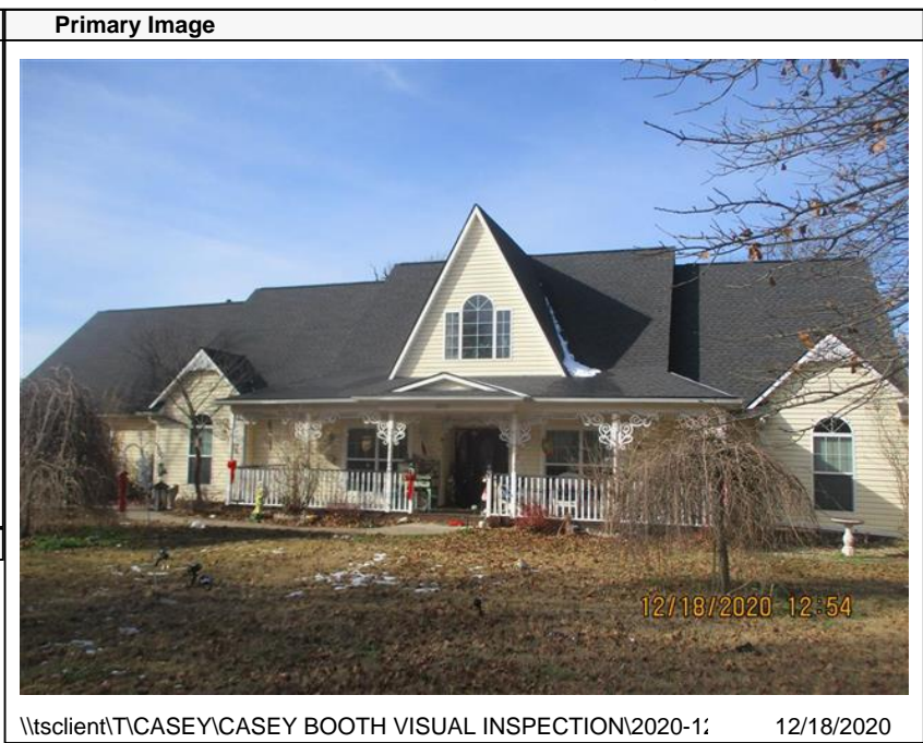
\\tsclient\TCASEY\CASEY BOOTH VISUAL INSPECTION\2020-1; 12/18/2020
