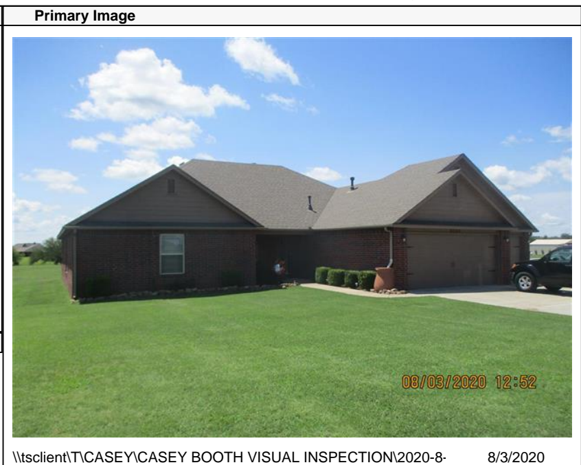
\\tsclient\TCASEY\CASEY BOOTH VISUAL INSPECTION\2020-8- 8/3/2020
