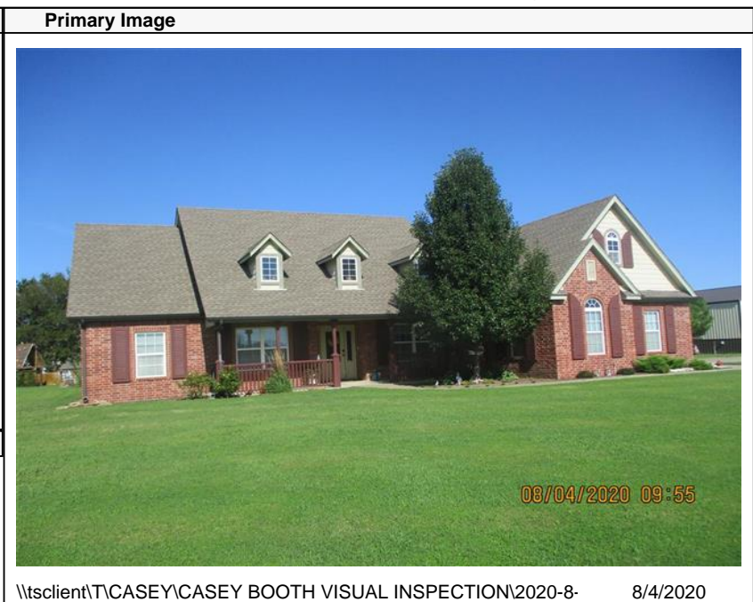
\\tsclient\TCASEY\CASEY BOOTH VISUAL INSPECTION\2020-8- 8/4/2020
