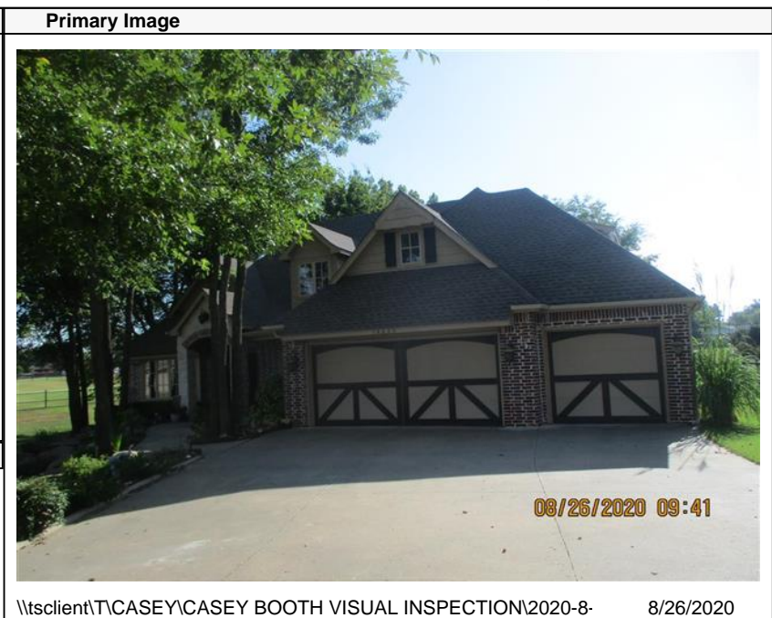
\\tsclient\TCASEY\CASEY BOOTH VISUAL INSPECTION\2020-8- 8/26/2020
