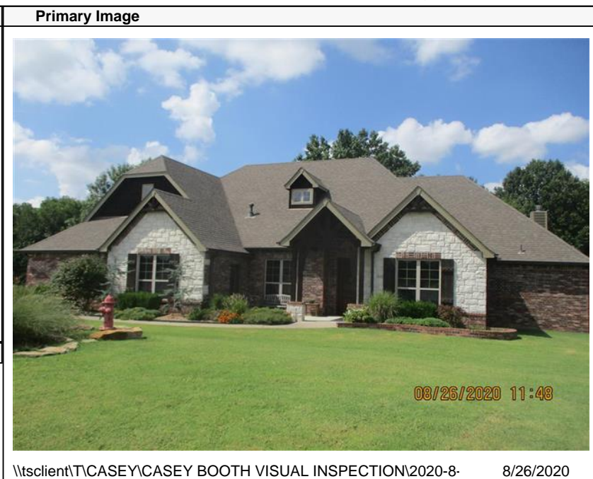
\\tsclient\TCASEY\CASEY BOOTH VISUAL INSPECTION\2020-8- 8/26/2020
