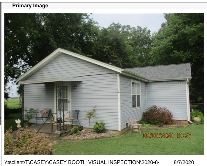
\\tsclient\TCASEY\CASEY BOOTH VISUAL INSPECTION\2020-8- 8/7/2020
