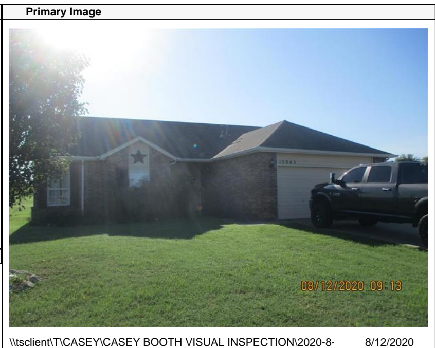
\\tsclient\TCASEY\CASEY BOOTH VISUAL INSPECTION\2020-8- 8/12/2020
