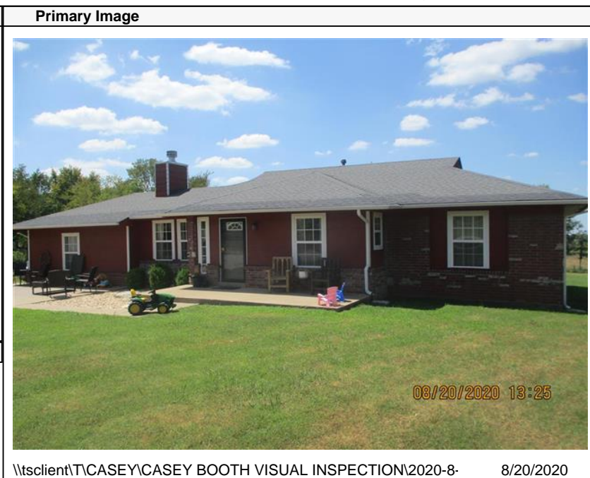
\\tsclient\TCASEY\CASEY BOOTH VISUAL INSPECTION\2020-8- 8/20/2020
