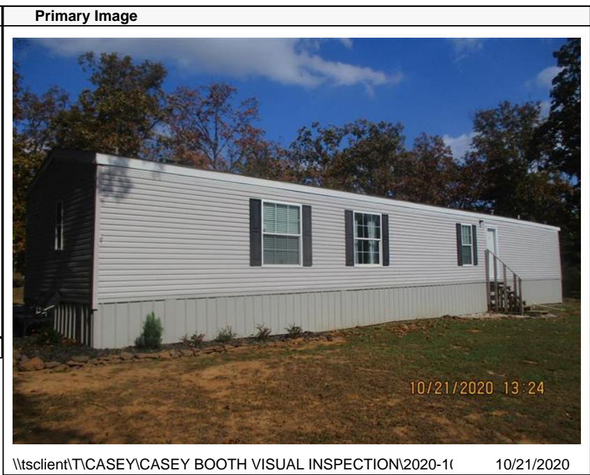
\\tsclient\TCASEY\CASEY BOOTH VISUAL INSPECTION\2020-1( 10/21/2020
