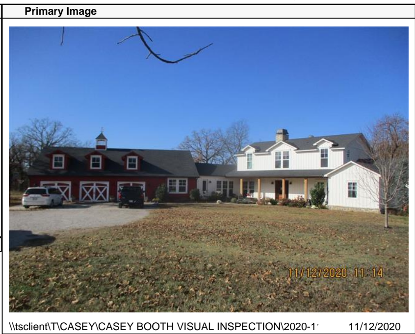
\\tsclient\TCASEY\CASEY BOOTH VISUAL INSPECTION\2020-1' 11/12/2020
