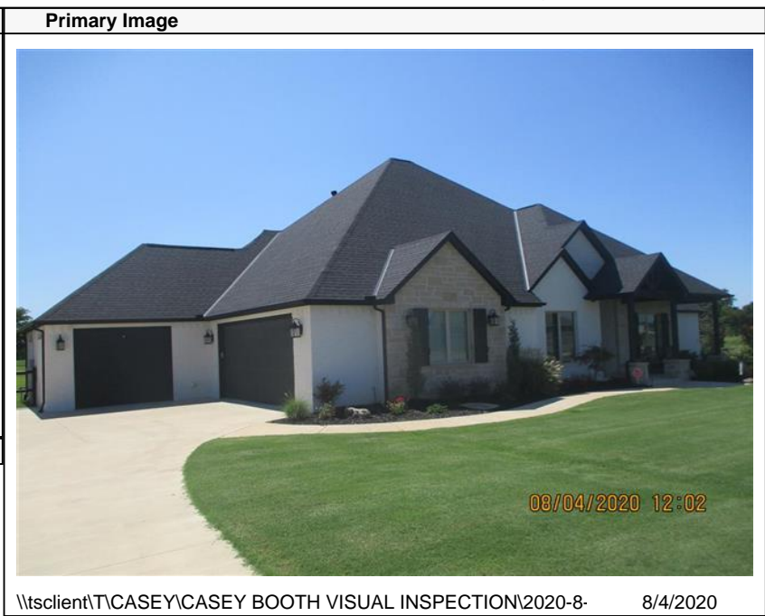
\\tsclient\TCASEY\CASEY BOOTH VISUAL INSPECTION\2020-8- 8/4/2020
