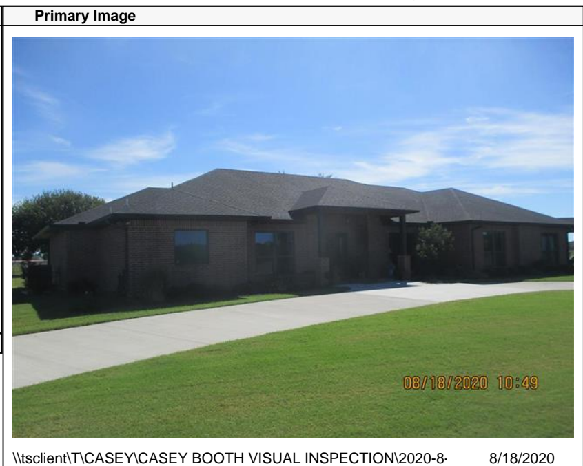
\\tsclient\TCASEY\CASEY BOOTH VISUAL INSPECTION\2020-8- 8/18/2020
