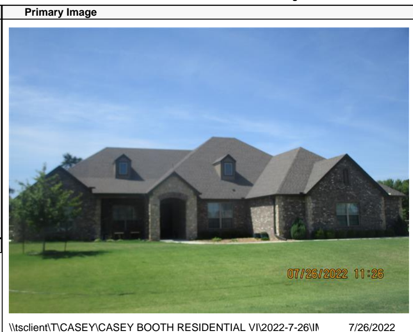
\\tsclient\TCASEY\CASEY BOOTH RESIDENTIAL VI\2022-7-26\ 7/26/2022
