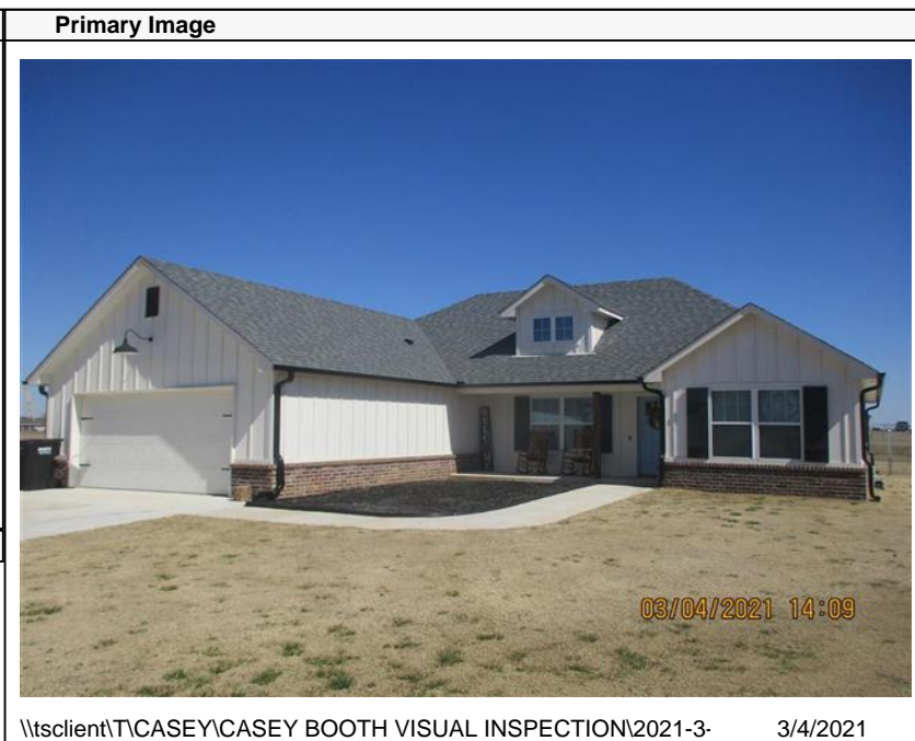
\\tsclient\TCASEY\CASEY BOOTH VISUAL INSPECTION\2021-3- 3/4/2021
