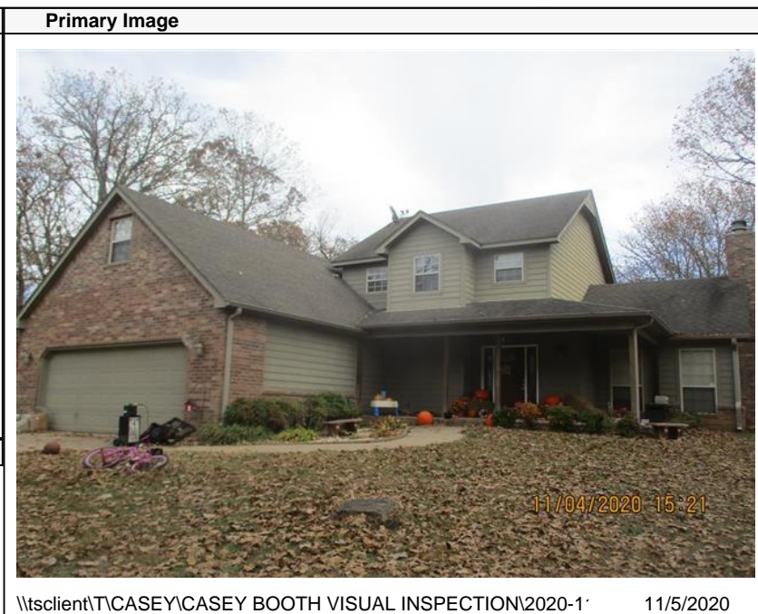
\\tsclient\TCASEY\CASEY BOOTH VISUAL INSPECTION\2020-1\ 11/5/2020
